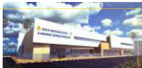
Aakari Training centre for maintenance of renewable energies - Rabat
